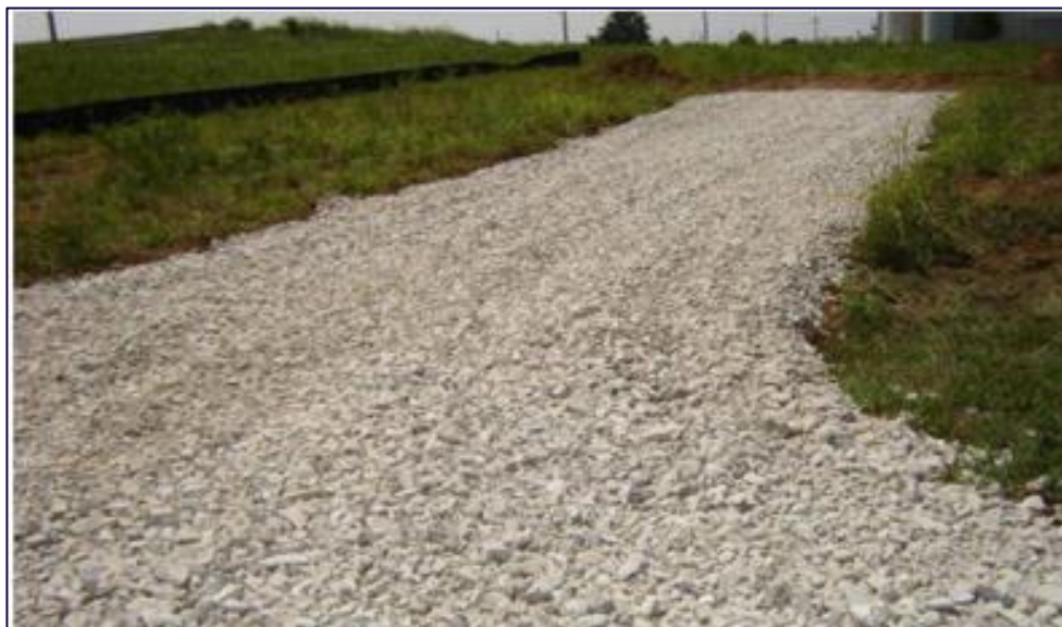
Figure 8.1: Temporary access track
